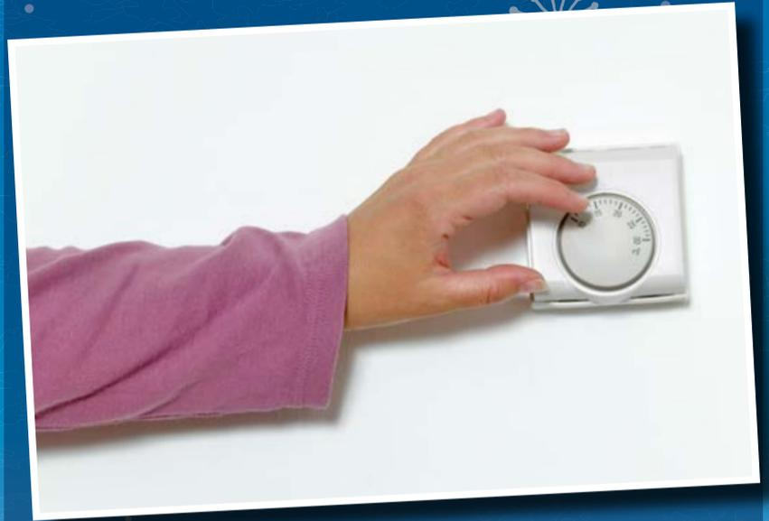
This is usually found in the living room or hallway and – for most people – it is recommended to be set between 18 and 21° C. The room thermostat will respond to the temperature in the room where it is situated. When the room is warm enough it sends a signal to the central heating pump to stop heating the radiators until the temperature drops below the set level. At this point they will come back on again.
