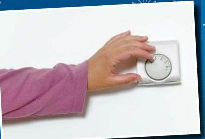
This is usually found in the living room or hallway and – for most people – it is recommended to be set between 18 and  $21^{\circ}$  C. The room thermostat will respond to the temperature in the room where it is situated. When the room is warm enough it sends a signal to the central heating pump to stop heating the radiators until the temperature drops below the set level. At this point they will come back on again.
