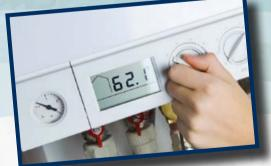
If your boiler is a 'combi' boiler, then the water is heated instantaneously when the hot water taps are switched on. For boilers which are not 'combi', the heated water also circulates through a coil in the hot water tank (also called an immersor), which in turn heats up the rest of the water in the cylinder to provide running hot water.
